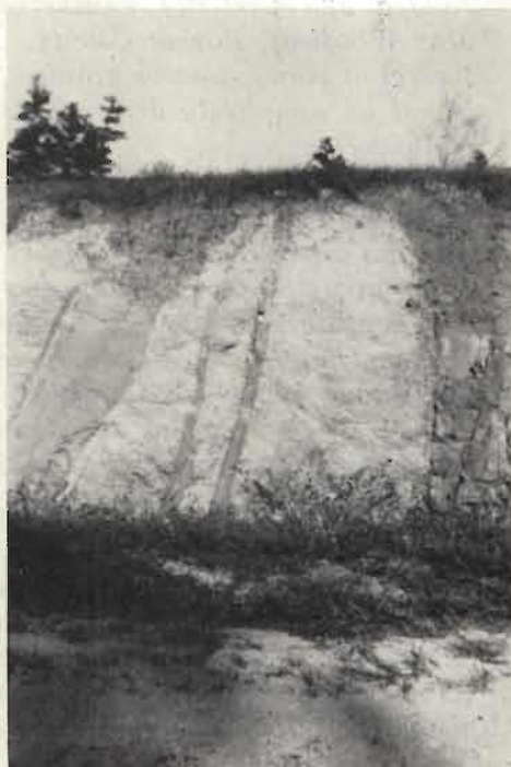
FIGURE 4.—Partially weathered granite (light) and diorite (dark) in road cut along U. S. Route 29, about 3 miles west of Thomasville, Davidson County.
