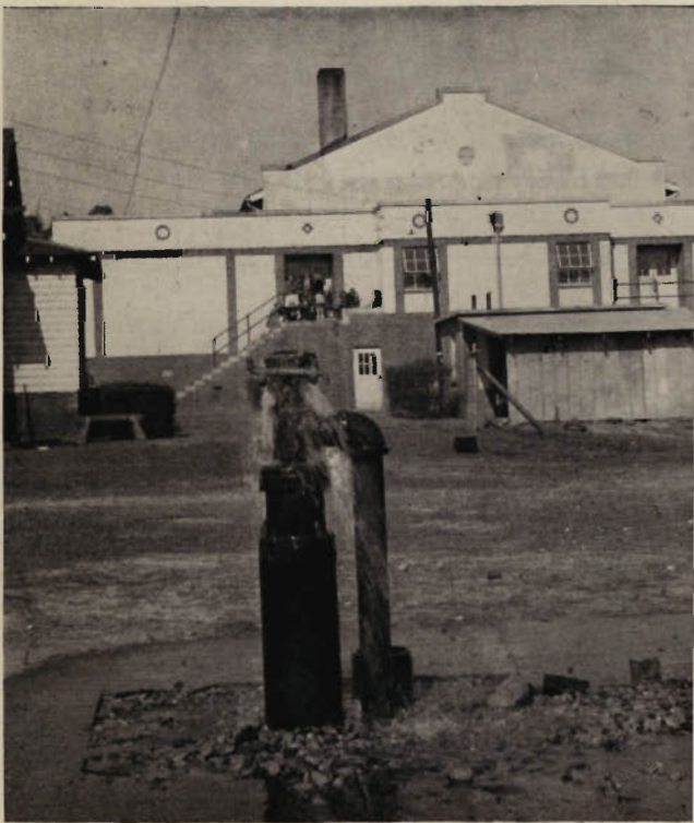
A.—Flowing well at Bullocks School in Wilson County. This well is drilled in granite and is 159 feet deep. When drilled, the flow was 60 gallons a minute, and the water would rise 12 feet above the surface.
