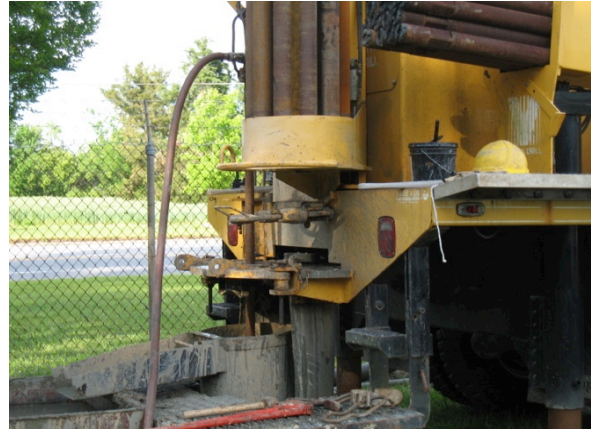
Pressure grouting using bentonite grout
