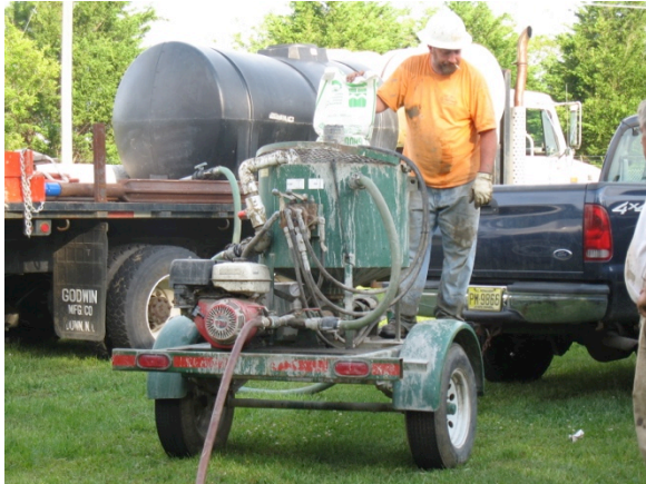
Pressure grouting using bentonite grout
