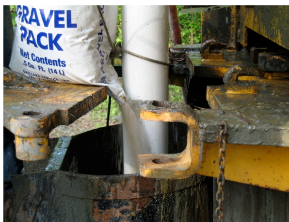
Gravel Pack Installation
