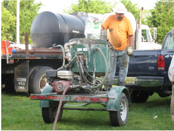
Pressure grouting using bentonite grout
