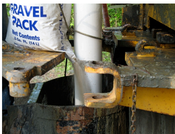
Gravel Pack Installation
