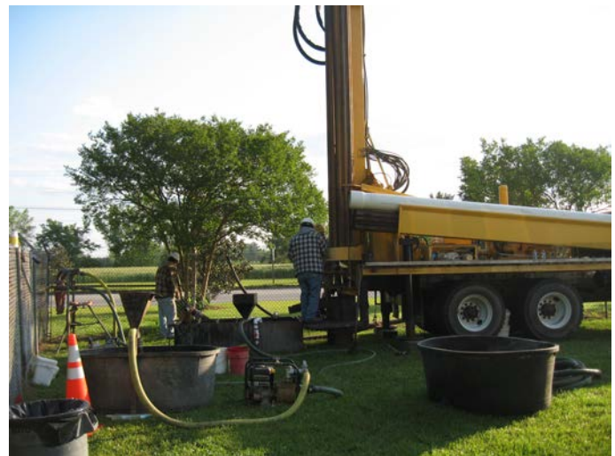
Well Installation Using Mud Rotary Drilling
