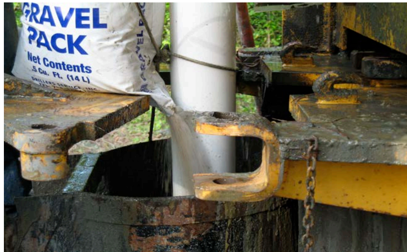
Installing Gravel Pack
