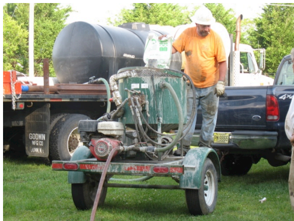
Pressure grouting using bentonite grout
