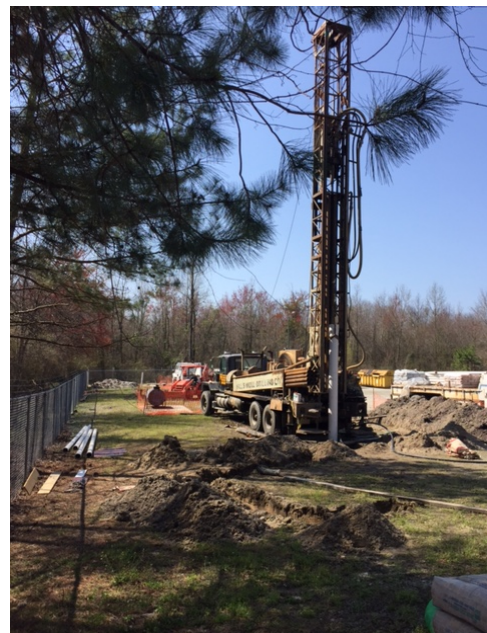
Well Installation Using Mud Rotary Drilling
