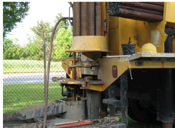
Pressure grouting using bentonite grout
