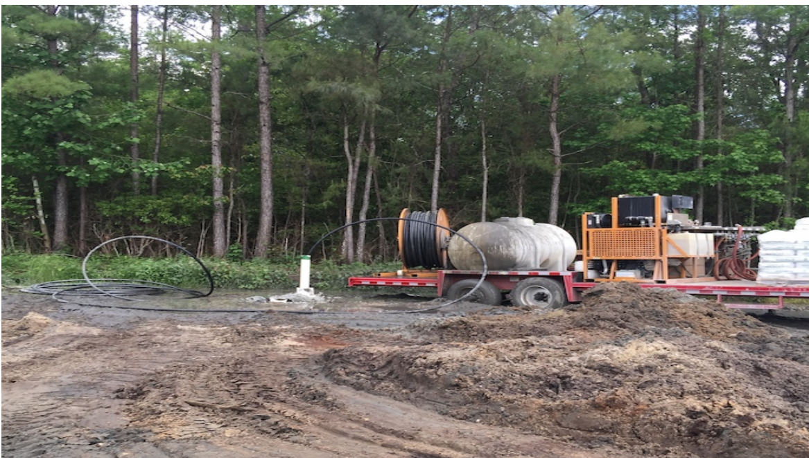
Well Development Holly Shelter Station, Z29N, Pender County
