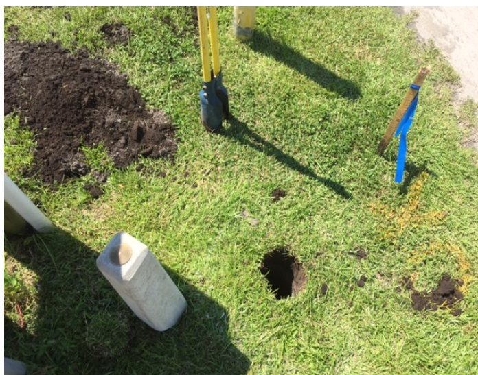
Monument Installation Montford Point Station, X24E, Onslow County
