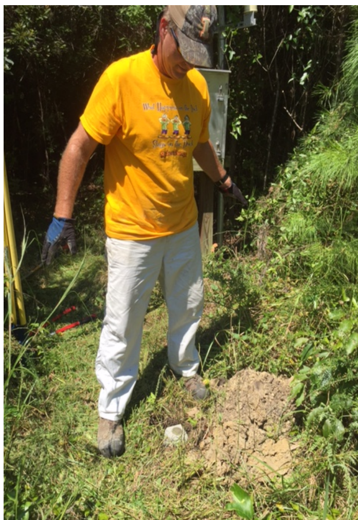
Monument Installation Ragged Point Station, X25U, Onslow County
