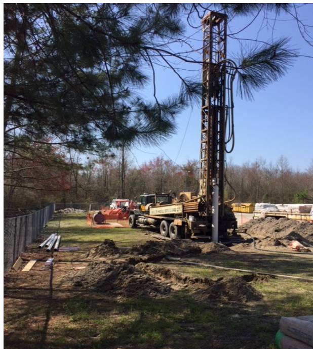
Mud Rotary Drilling Calypso Station, S33C Duplin County
