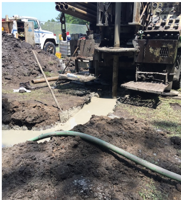
Mud Rotary Drilling Castle Hayne Park Station, CC30E New Hanover County
