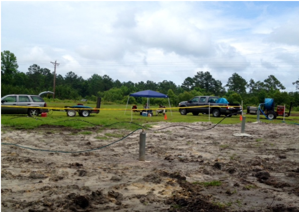
Well Development Nakina Station, EE390, Columbus County
