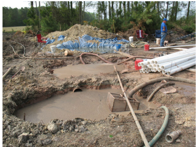
Mud Rotary Drilling using Mud Pits Nakina Station, EE 390, Columbus
