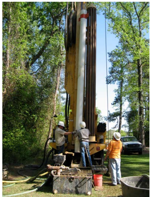
Well Installation, Ivanhoe Station, Y 34P, Sampson County
