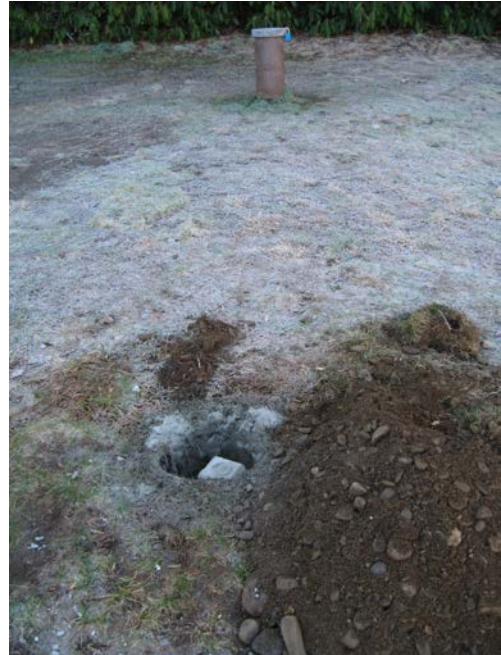
Installed Monument Woody Creek Station, M 93L, Haywood County
