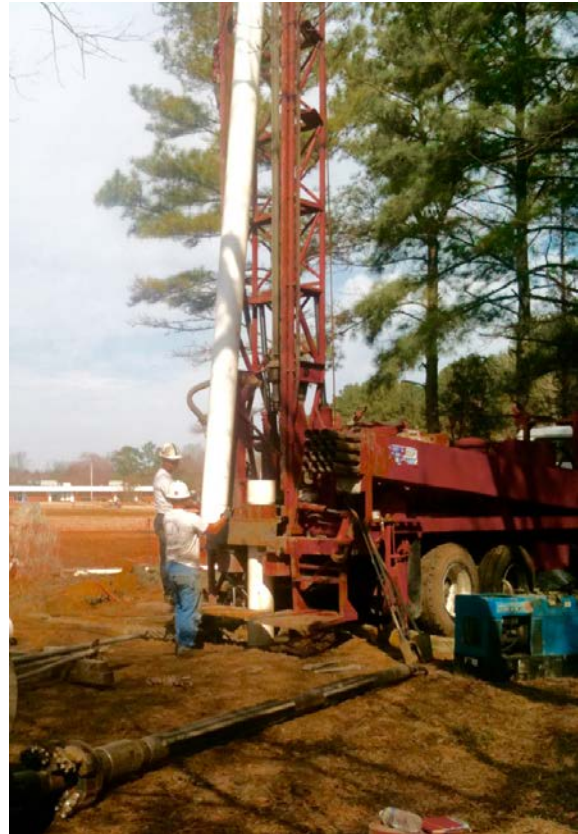
Well Casing Installation Rose Hill Station, V 32V Duplin County
