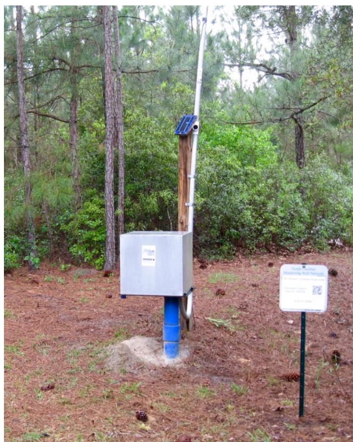
Solinst Telemetry System Clarendon Station, DD 42N, Columbus County
