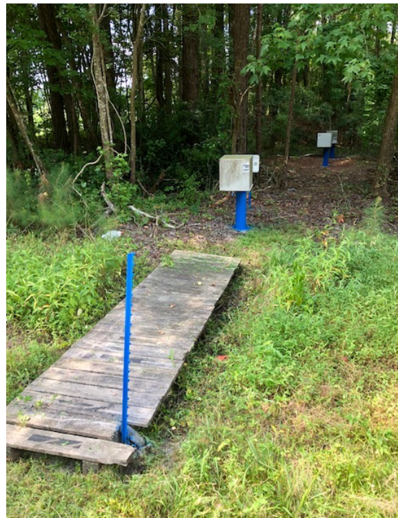
Hwy 102 Station O 21Q, Pitt County
