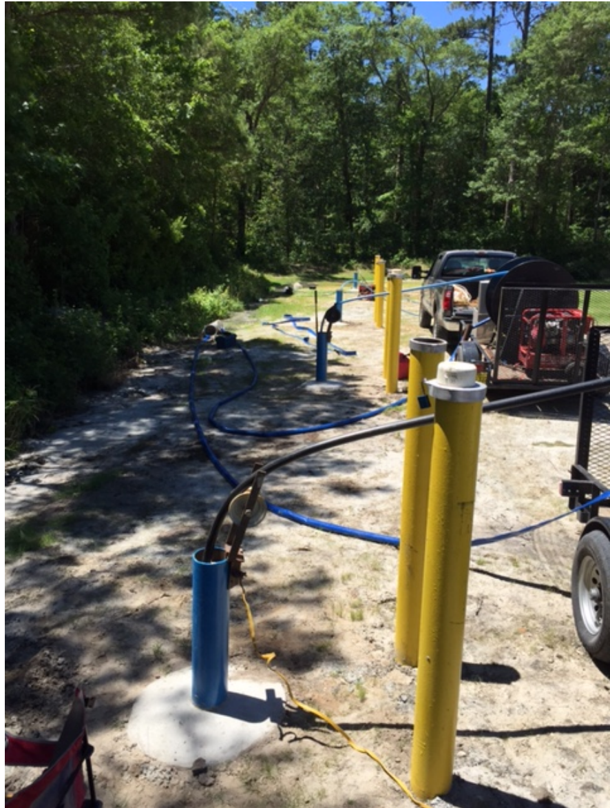
Well Development Holly Shelter, Z 29N, Pender County
