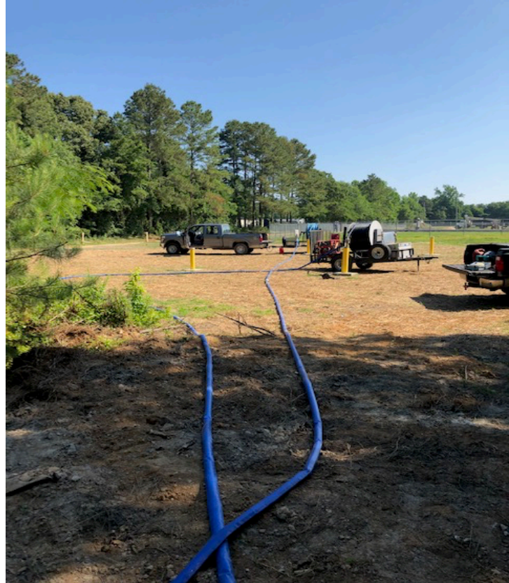
Well Development Clinton Station, U 35I, Sampson County
