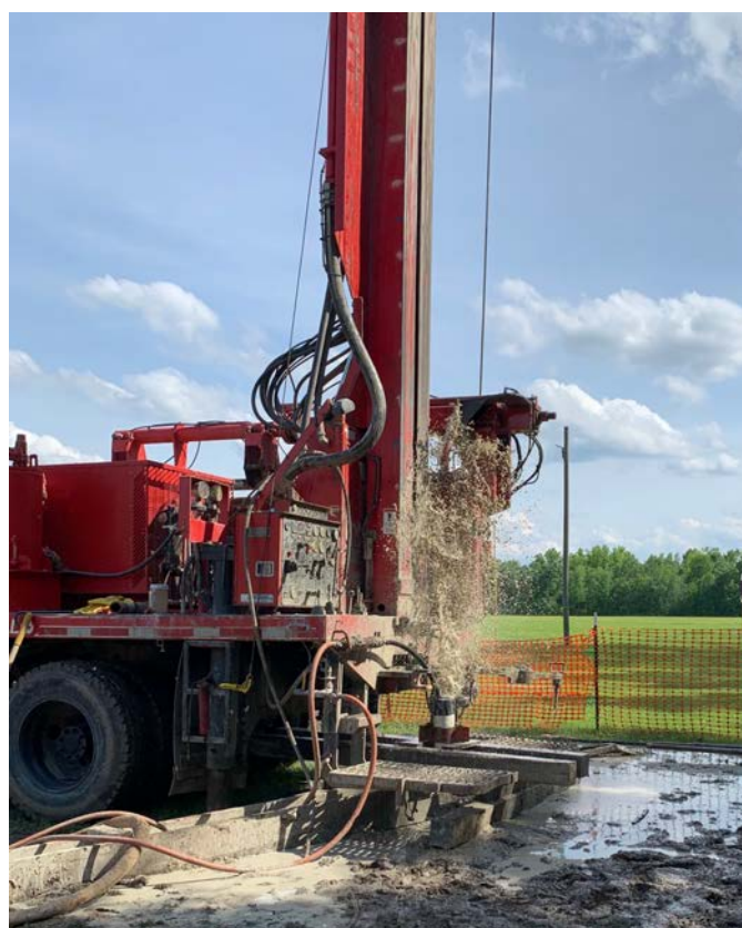
Well Development Chinquapin Elementary School Station W 29D, Gates County
