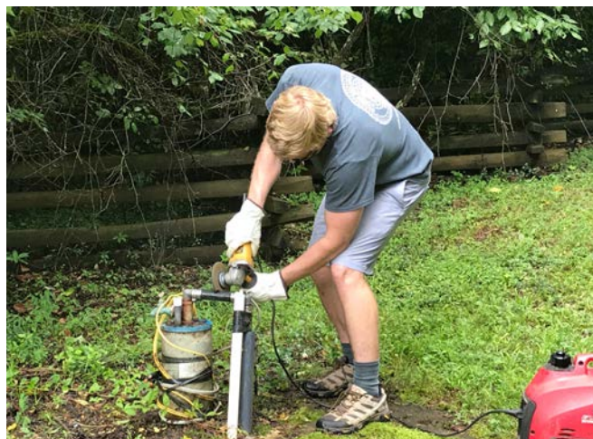
Pump Removal Ivy Bluffs Access Station, E 62U, Yadkin County
