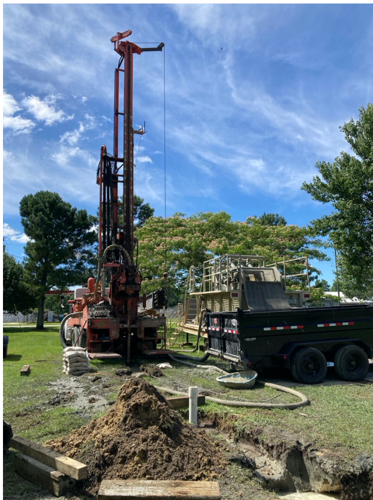
Well Installation DF Walker Elementary School (G 15R) Edenton, Chowan County, NC
