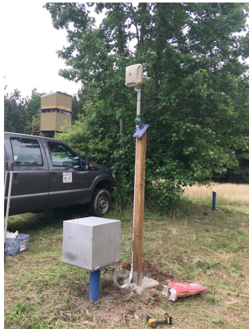
STS Repair Lewiston Station (H 22I), Bertie County,
