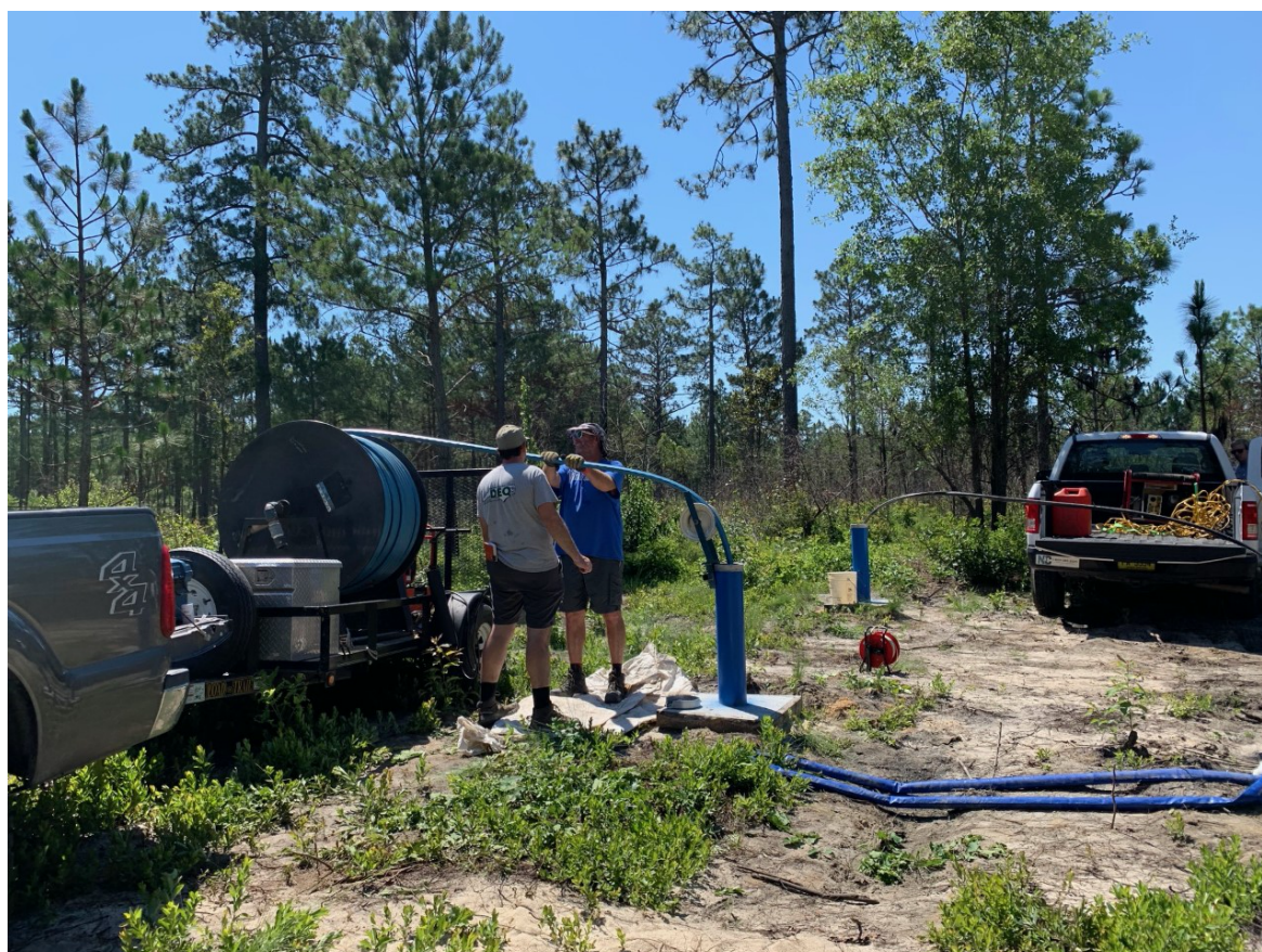
Well Development Pondberry Bay Station (U 37D), Sampson County, NC
