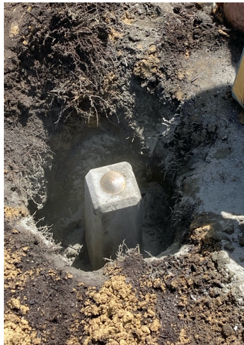
Monument Installation DF Walker Elementary School (G 15E) Edenton, Chowan County, NC
