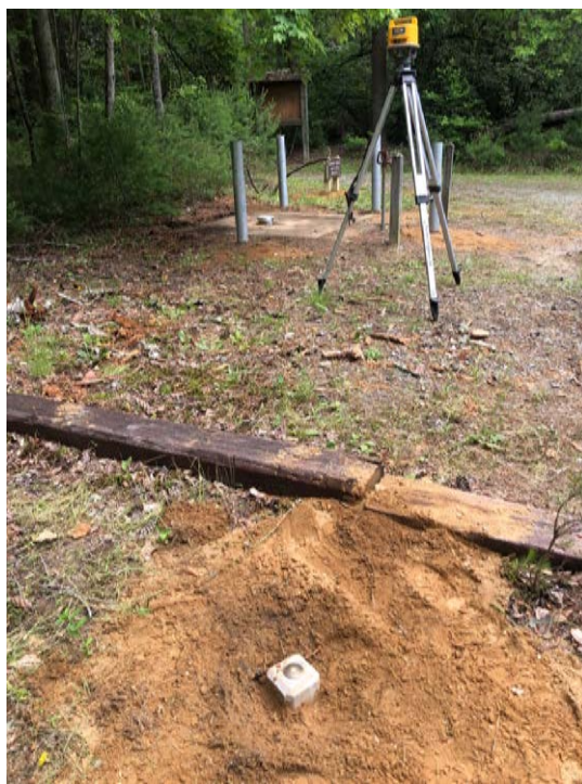
Monument Installation Stone Mountain Station, G68X Wilkes County, NC
