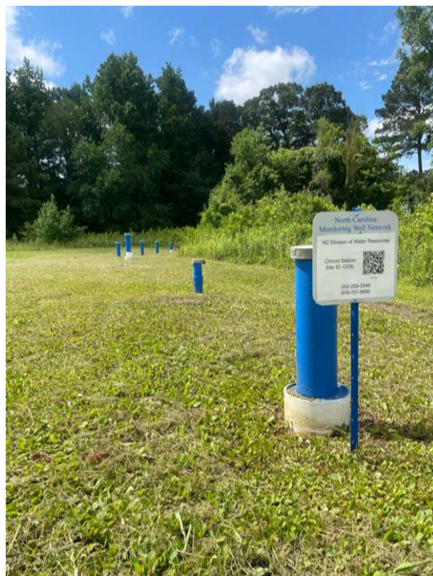
Chicod Monitoring Station, O23L Pitt County, NC
