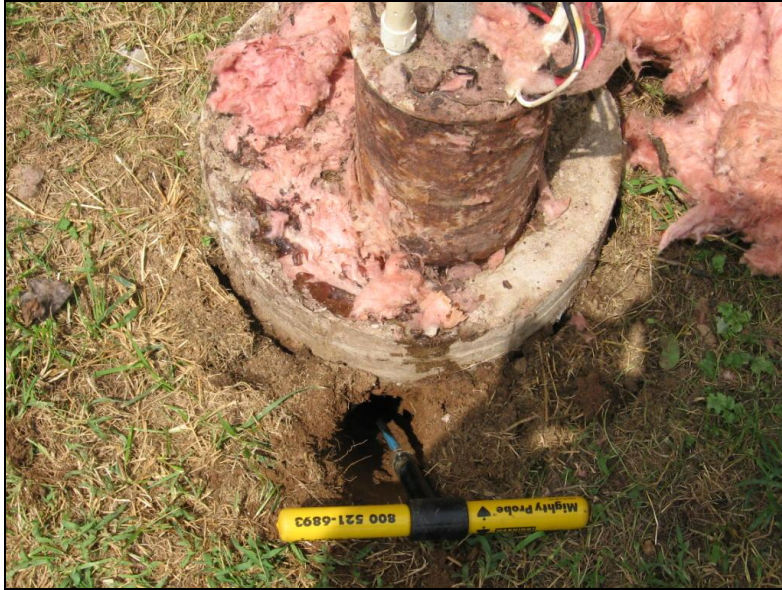
Figure 7. Example of improperly constructed, un-grouted well in survey area.
